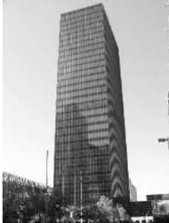
Figure 1. Exterior of Building
