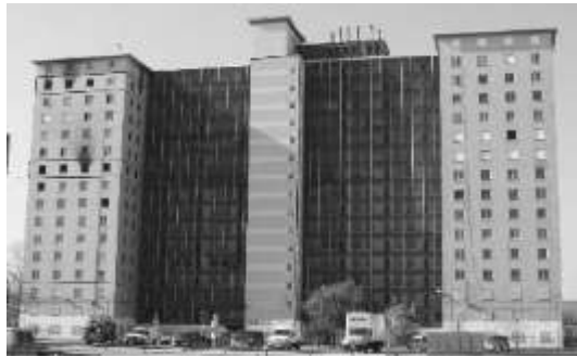
Figure 8. Front Elevation of the building.
